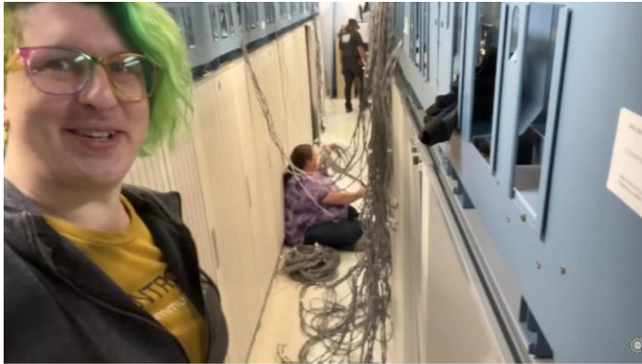
Volunteers Sarah and Angela remove complex cabling
