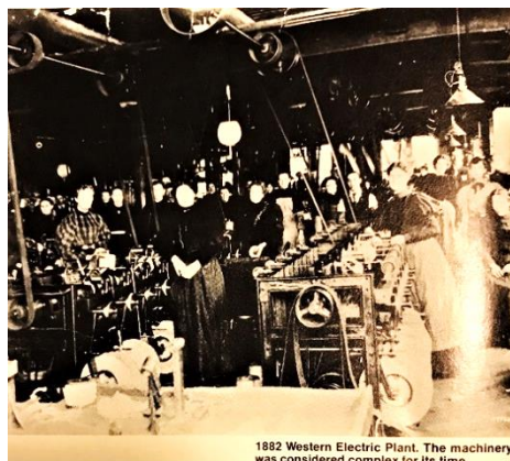
1882 Western Electric Plant. The machinery was considered complex for its time.
