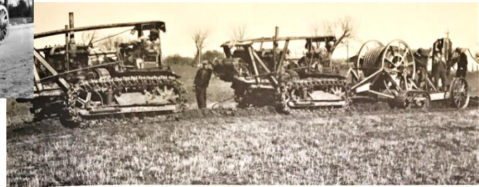
1930. Construction crews bury cable between Kansas City and Joplin.
