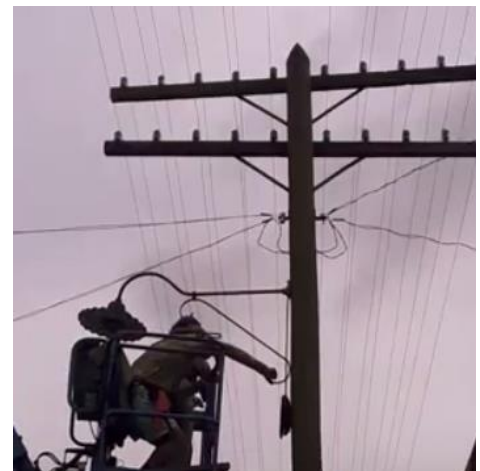
Historic street lighting installed
