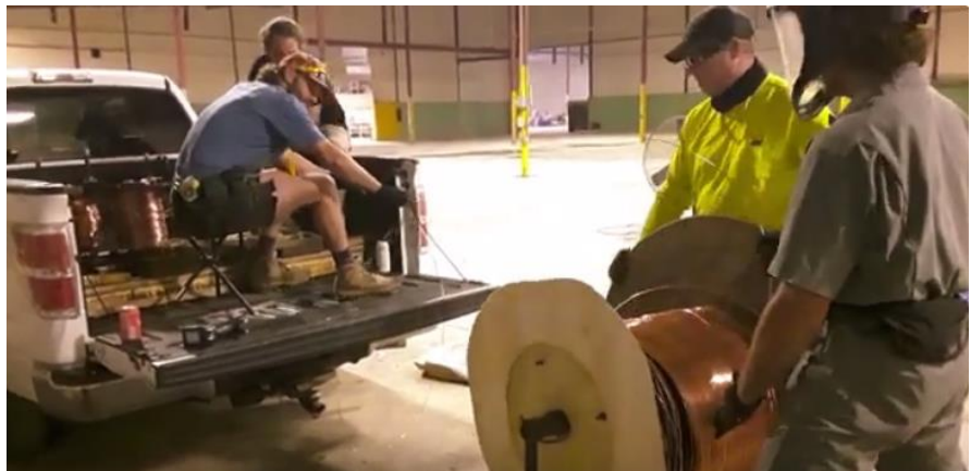
Spooling wire on a re-created device to efficiently hang four lines
