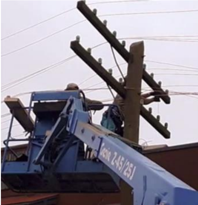
Hanging wire four conductors simultaneously
