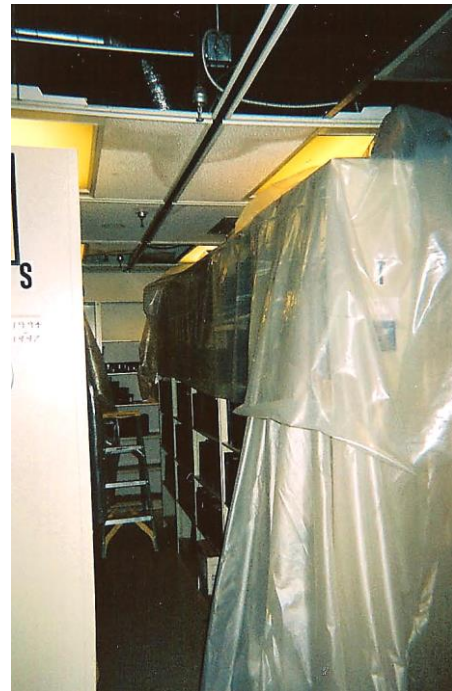
The directory room with sheets of plastic over shelving.
