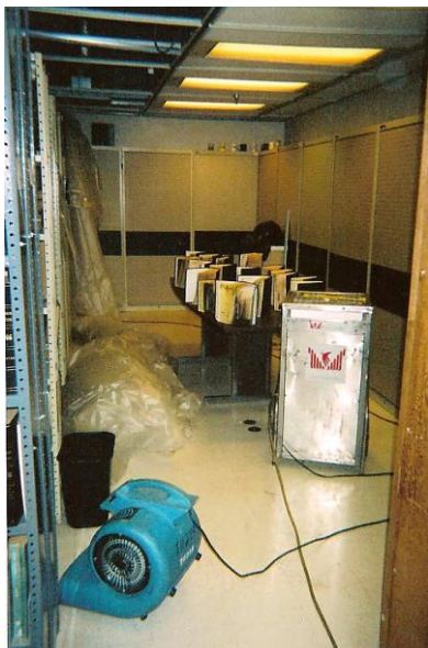
Directory room with fans and dehumidifier.
