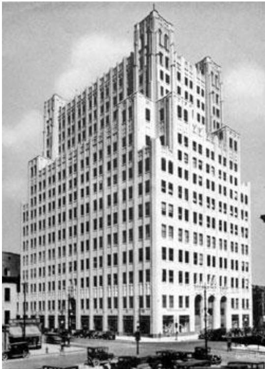
The telephone building at 931 14th St, Denver, Colorado. (THG archives)
