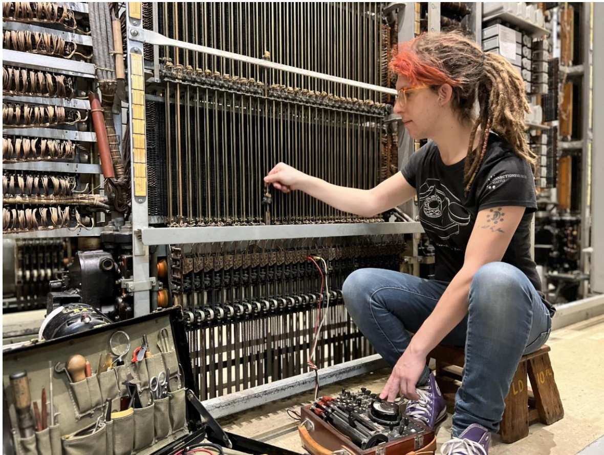
Subject matter expert (and panel switch caretaker) Sarah Autumn of THG's Connections Museum is shown working on a section of the switching system.
